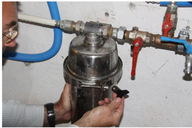
**Remove the old filter cartridge (which can be thrown in the trash)**
