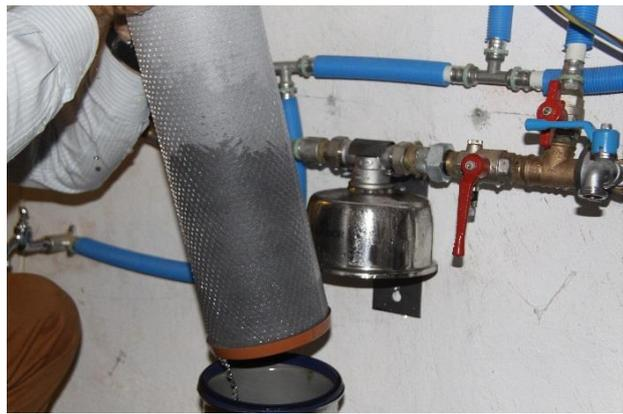
**Discard the water at the bottom of the Biofilter housing (the water may be black due to the active carbon coming out of the filter that is no longer under pressure or brown if there is oxidation in the pipes. galvanized from the city water distribution company = iron oxide) & wash the inside of the half-case, the 2 black rubber gaskets and the blue plastic ring:**
